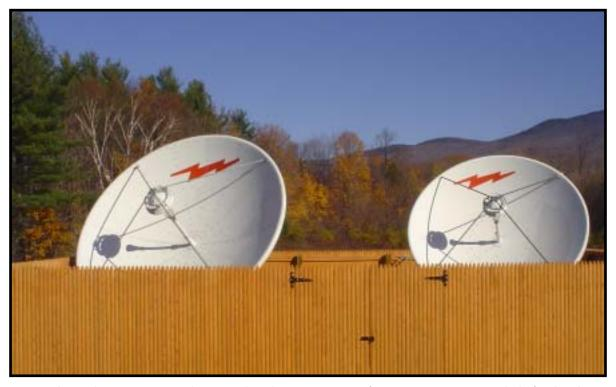
CVC Paging is pleased to announce the completed construction of our new paging up-link facility located at our corporate offices in Rutland, VT. The up-link facility is 100% redundant and features Andrew 4.6 and 3.7 meter earth station antennas. The implementation of our redundant up-link facility provides satellite redundancy, increased network efficiency and enhanced command and control capabilities.
